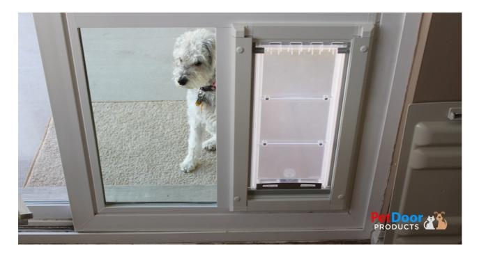
The best efforts of homeowners who invest in energy-efficient windows and doors can be undermined by aging or poorly designed pet doors. In fact, many lower-quality dog doors are sources of continuous major heating and cooling losses. Inferior doggie doors can also be extremely inefficient for protection from blowing dust.
