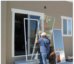
Step (4) Remove Old Glazing Tape Around Inside Edge of Sliding Door Frame
